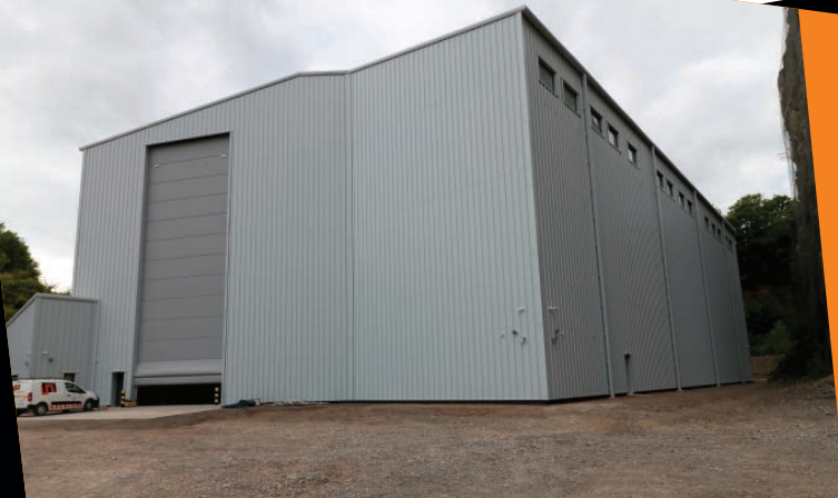
New Warehouse Facility - Wells
