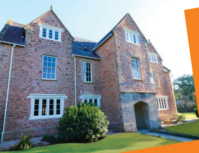
Refurbishment of a Grade II listed building for Wells Cathedral
