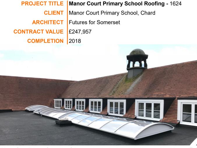
Manor Court Primary School is a fully operational school situated within a residential area off of Duck Lane in Chard. Areas of flat roof on Block B were in poor condition and poorly detailed which resulted in water ingress into the building.
