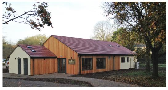
The project comprised construction of a detached single storey building, traditionally built with concrete floors, block work cavity walls, trussed roof and associated ground works, including drainage.
