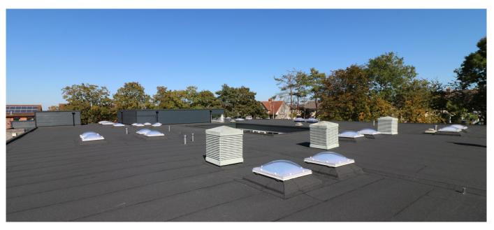
The works comprised of the re-roofing of the school building Block A, along with the replacement of the existing roof lights, uplifting the perimeter edge, roof cowls and replacement and extension of the existing cladding to the perimeter of the roof and upstand to the high level roof areas.
